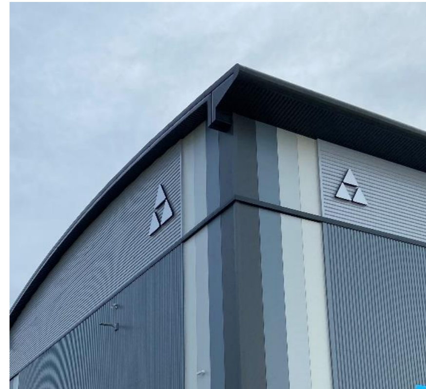
Fig 57. Illustrative building signage.
