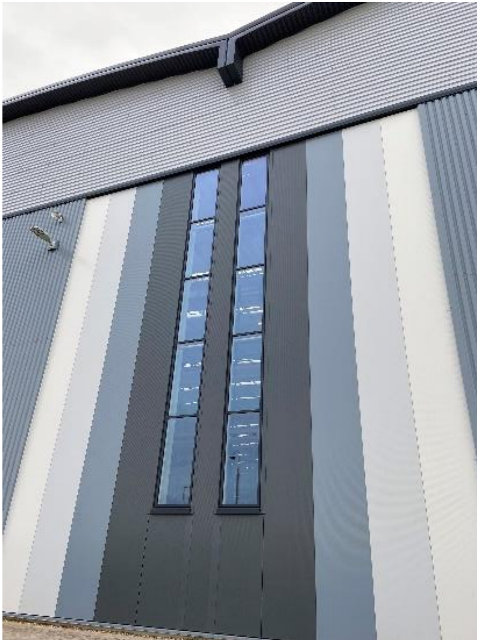
Fig.46 Application of material and colour
